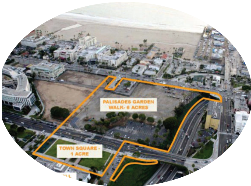
PRE-CONSTRUCTION SITE FOR TONGVA PARK https://inhabitat.com/high-line-park-designer-completes-new-tongva-park-in-santa-monica/tongva-park-james-corner-field-operations-5/
