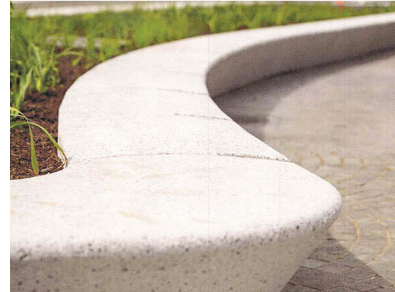
Cast-in-Place Concrete Benches with Steel Reveal Joints
