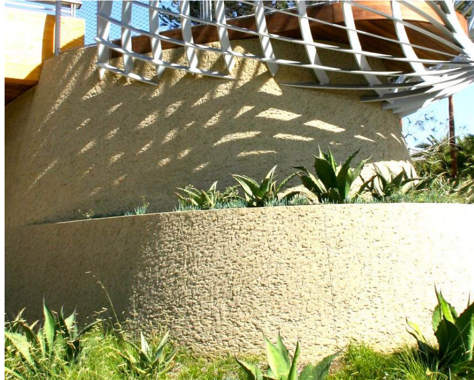
Rough Concrete, Steel Cage, and Wood Platform
