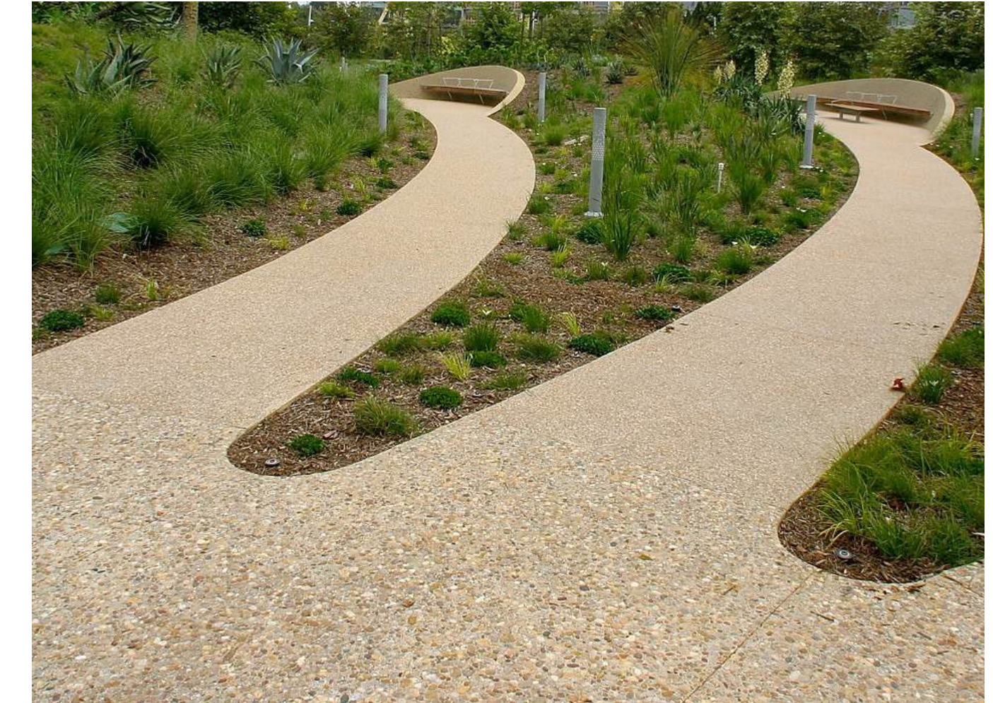
Visible Aggregate Concrete Walkways
