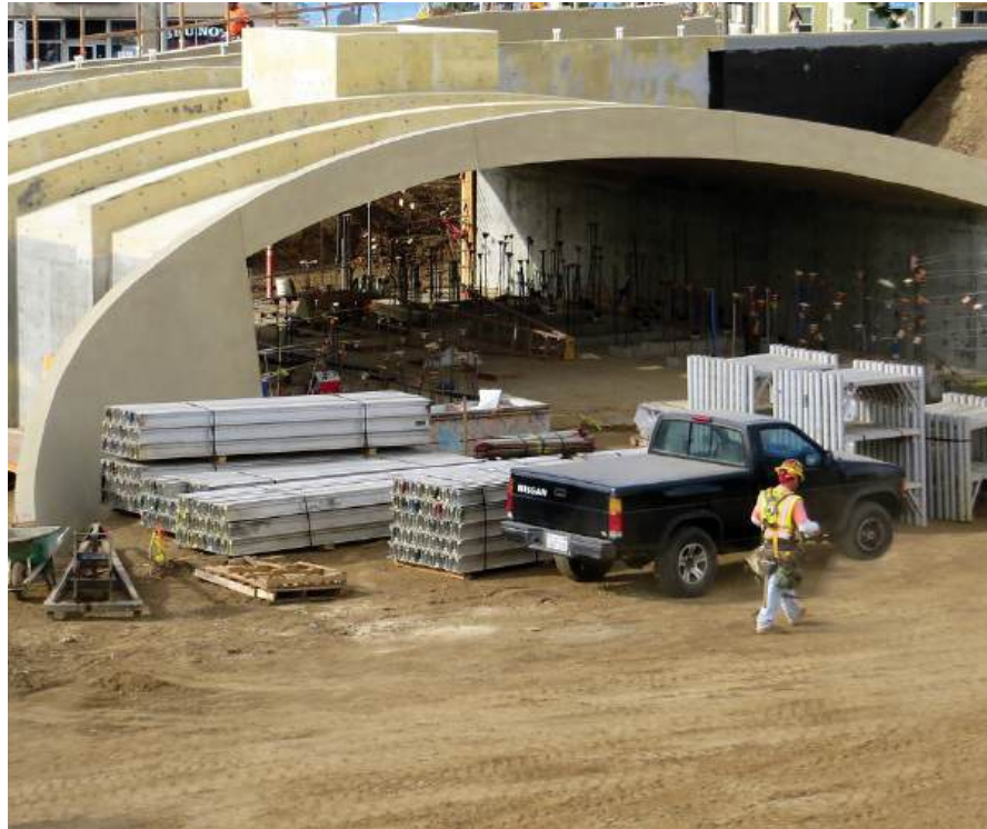
Post-Tension Concrete for Bathroom Structure
