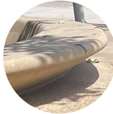
Concrete benches and retaining walls
