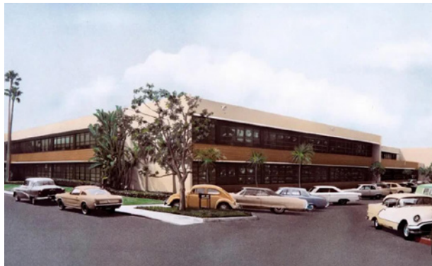
The previous Rand Corporation Building 1965
