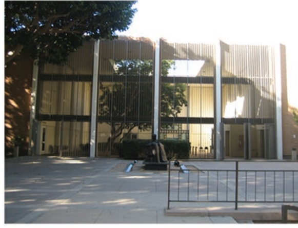
3 - OPEN WEAVE FACADE ALLOWS FOR WIND & NOISE
