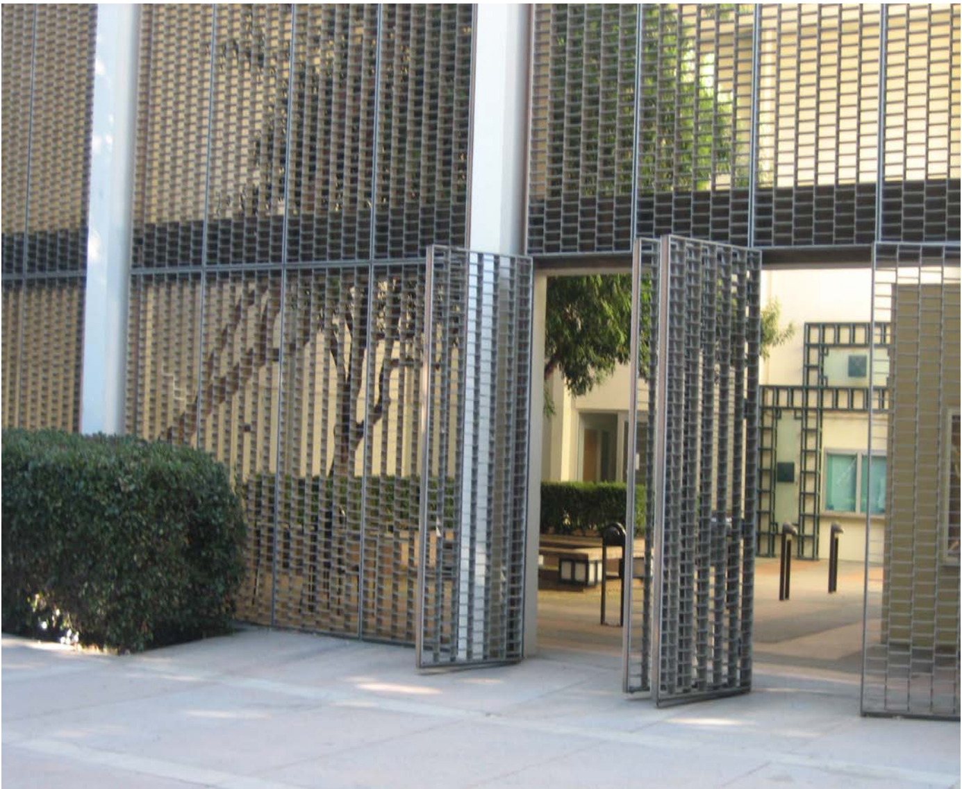
FRONT FACADE LOOKING INSIDE BUILDING
