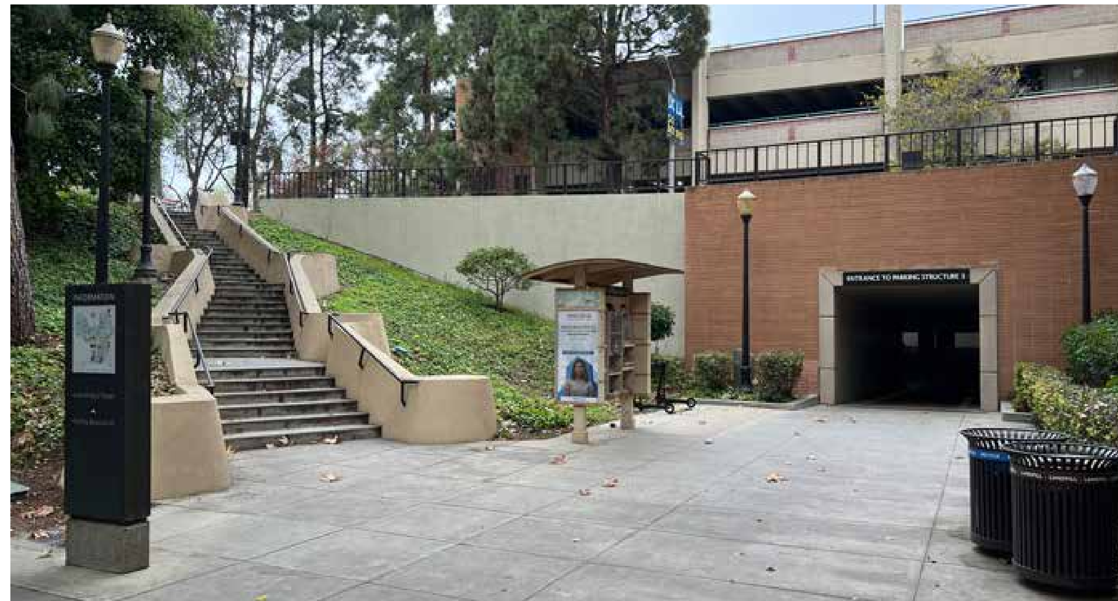
North Facing Tunnel to Parking Structure
