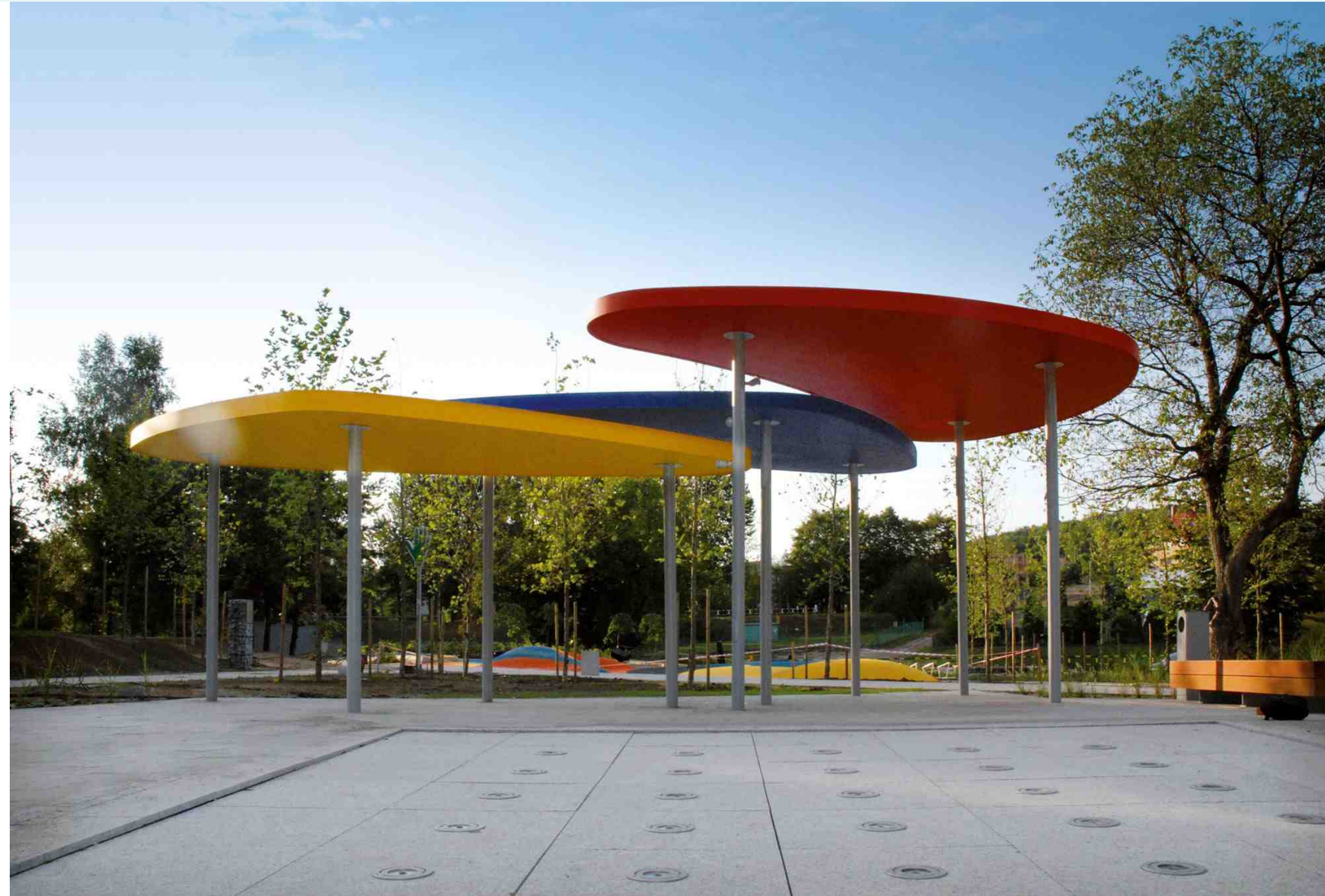
Multi-function covered structure in primary colors, tilted to direct drainage.
