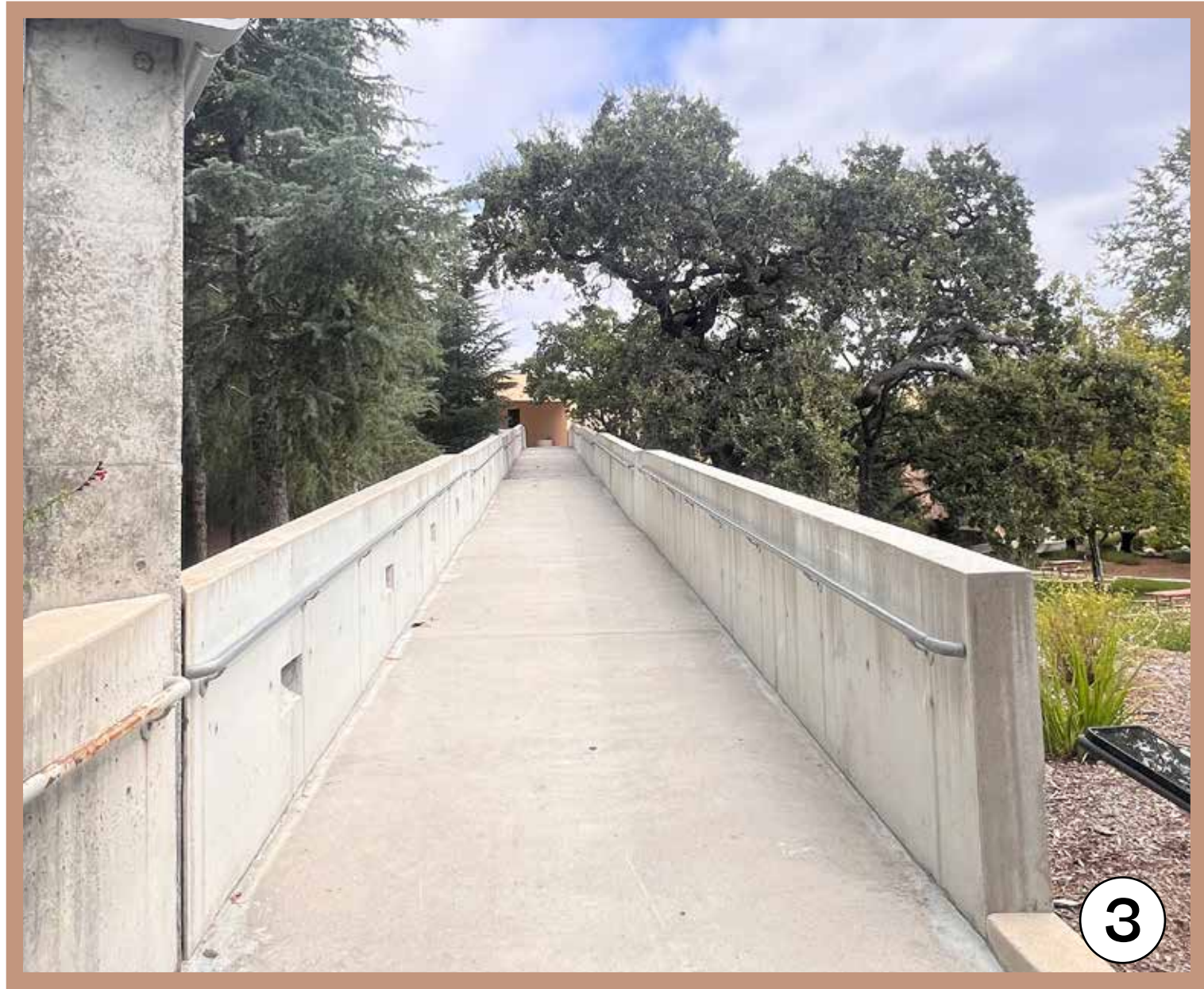
Pedestrian Bridge The elevated bridge provides an important connection across the site but functions primarily as a circulation route. Limited seating, planting, and moments of pause reduce the overall pedestrian experience.
