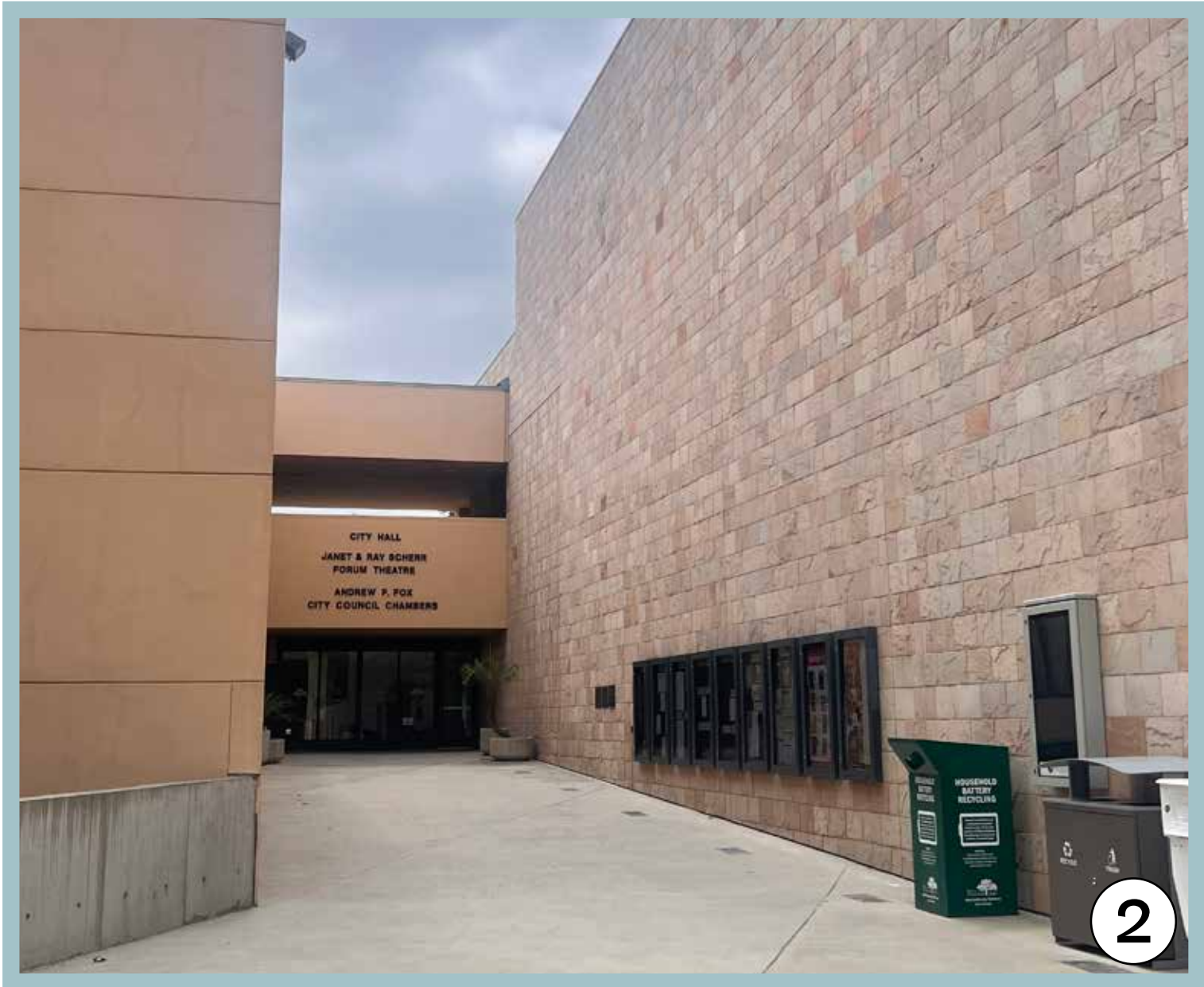
City Hall Entrance Access is provided via an elevated walkway, creating an indirect and understated approach. The entrance lacks visual prominence and an inviting pedestrian sequence.
