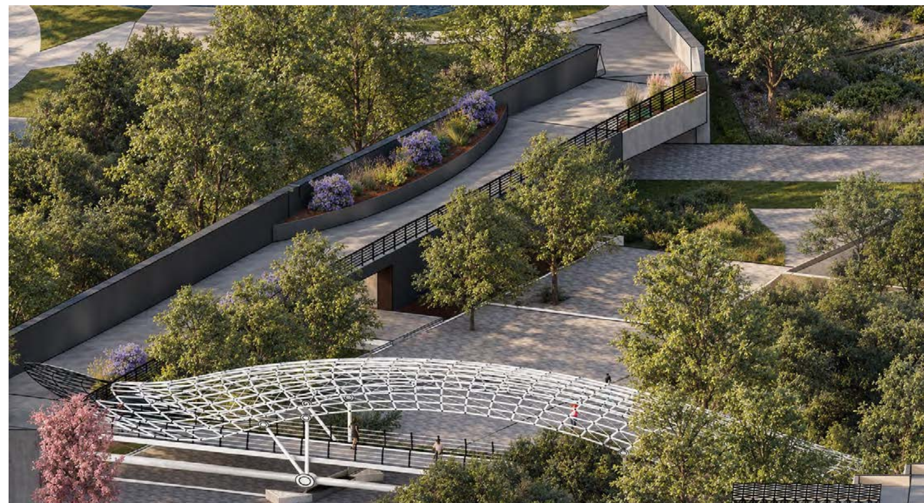
BRIDGE + ADA RAMP FROM THE LAKES
