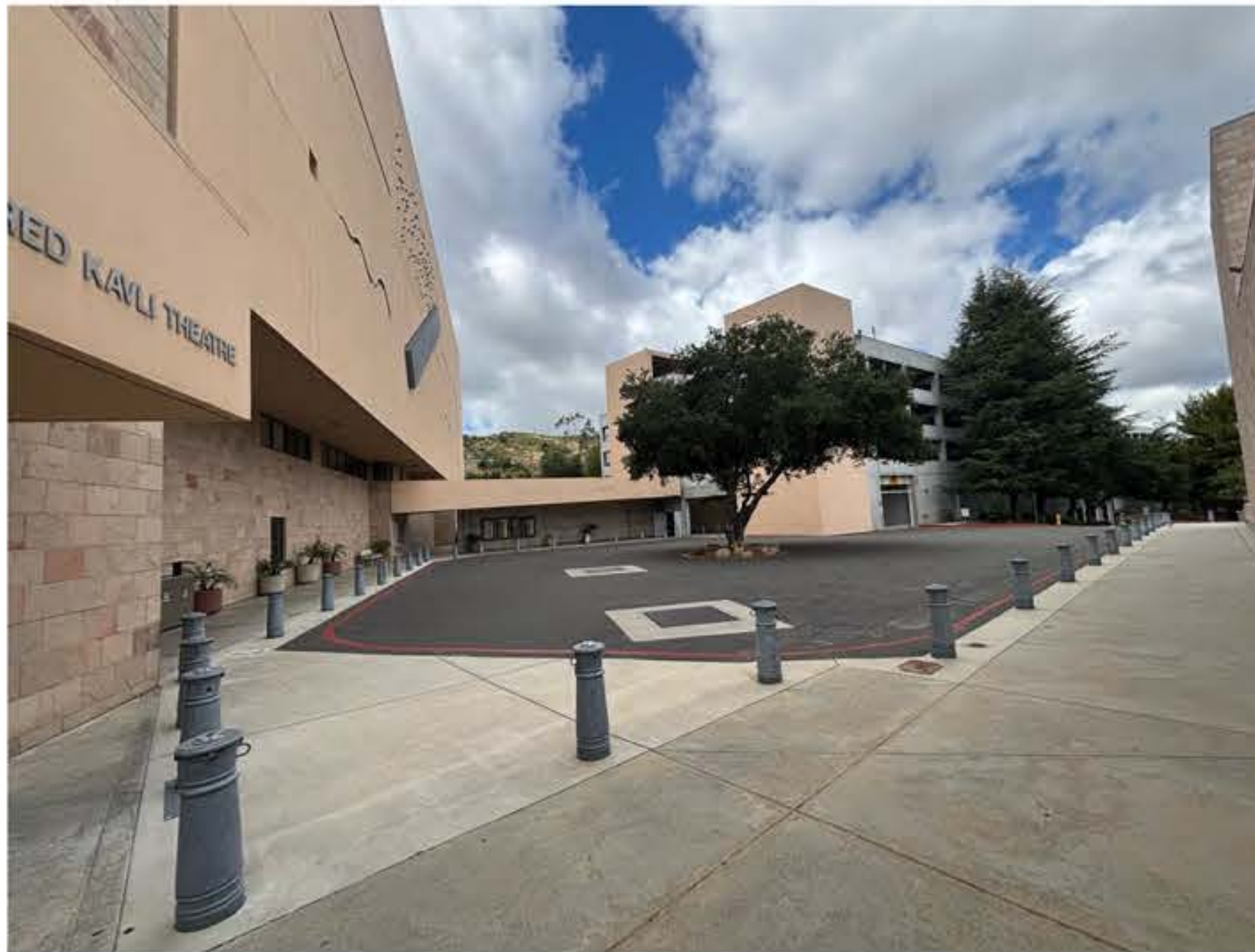
DROP OFF AREA AT ENTRANCE TO THEATER PARKING STRUCTURE IN DISTANCE
