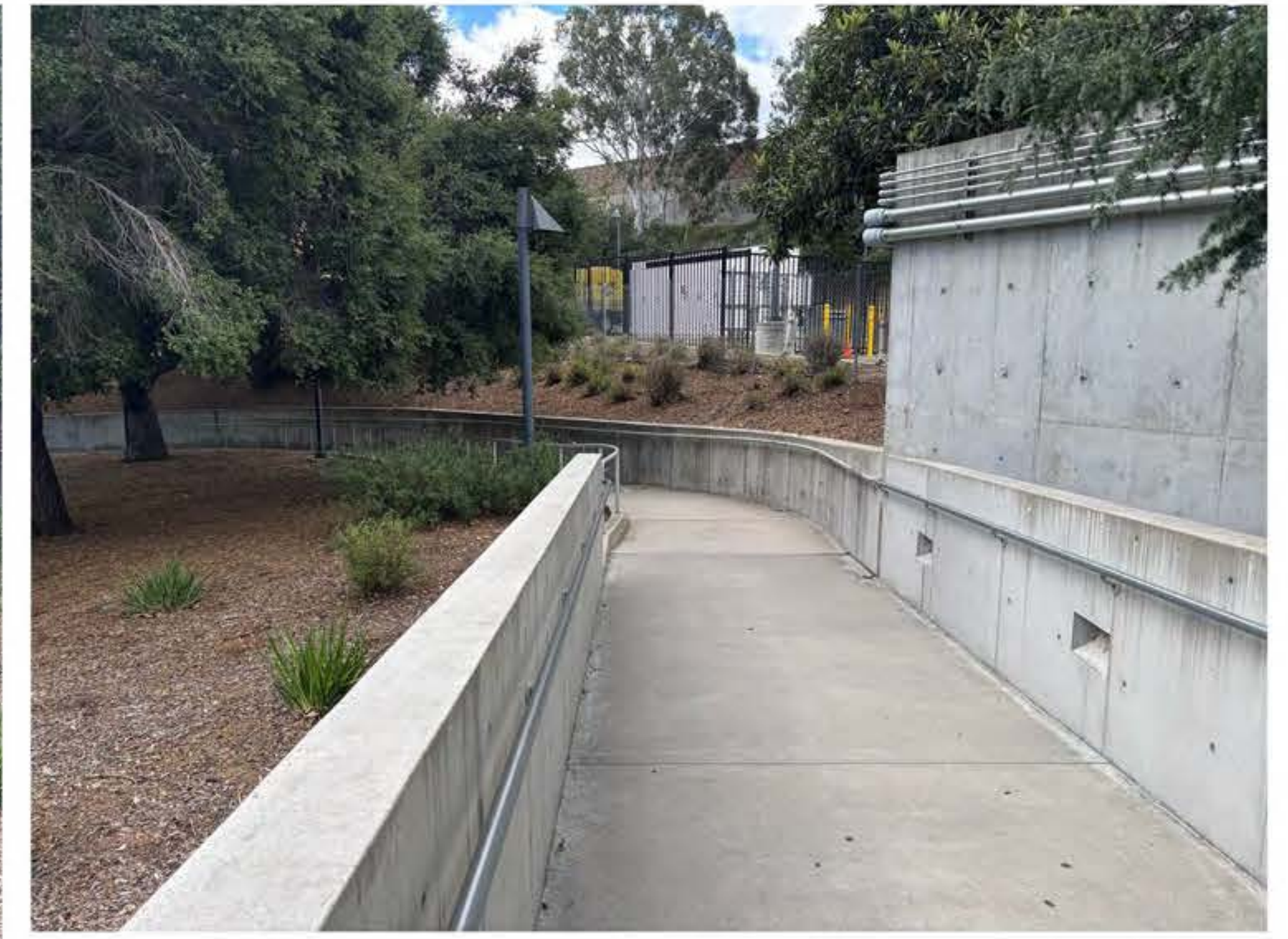
ACCESS RAMP FROM CIVIC CENTER DOWN TO LOWER AREA ON EAST SIDE OF GROUNDS.
