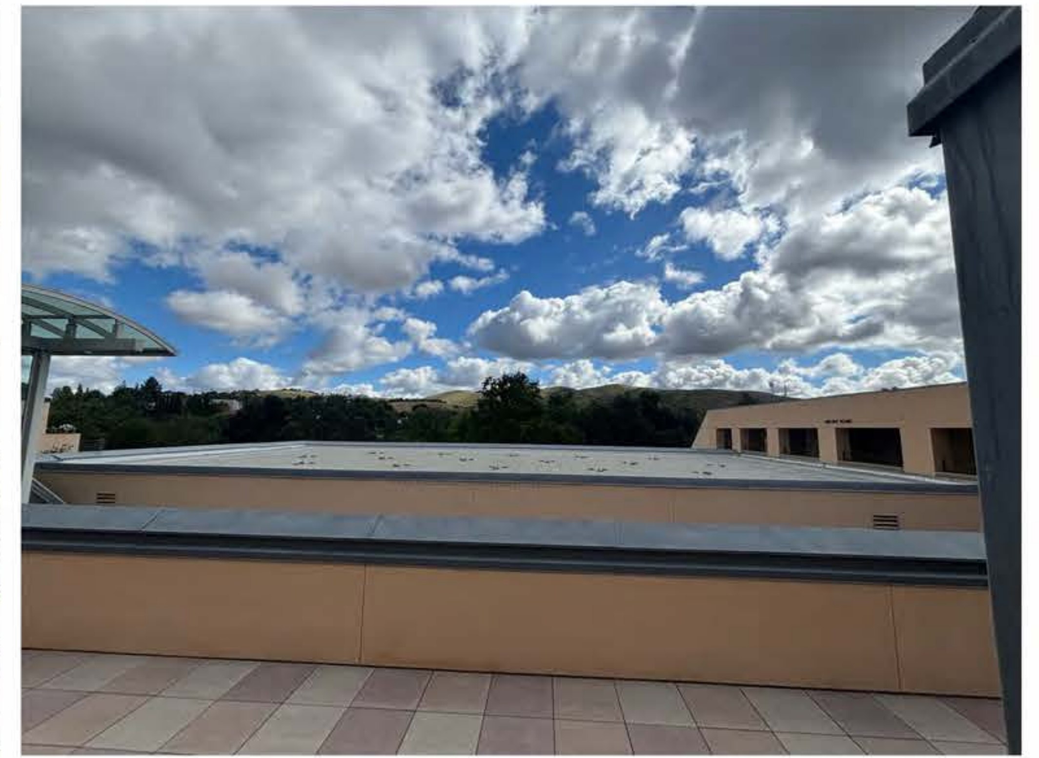
VIEW NORTH OVER DEFUNCT ROOFTOP WATER FEATURE WITH THE SANTA MONICA MOUNTAINS IN THE BACKGROUND
