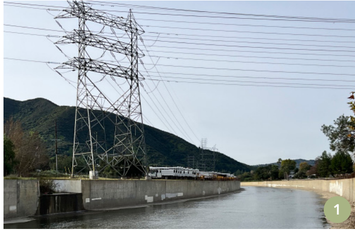
Large power lines through the park and along the LA River; concrete channel
