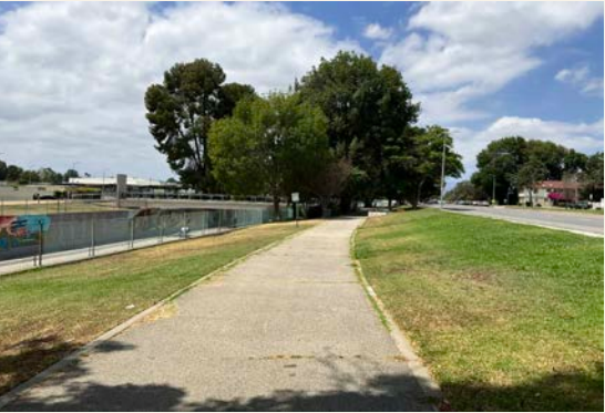
THE PEDESTRIAN PATH ALONG COLDWATER CANYON AVE. NO VISUAL OR SOUND BUFFER EXISTS BETWEEN THE ROAD AND THE PARK SPACE.
