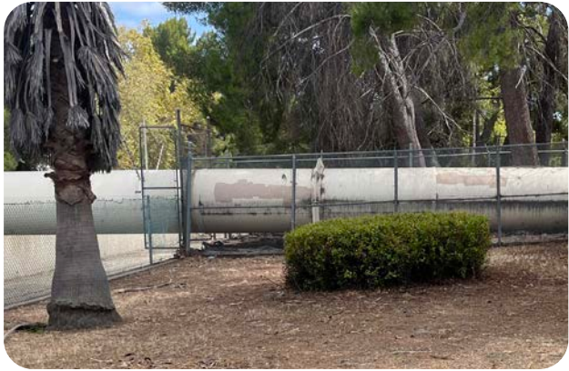
Large utility water line crosses over the wash and disrupts views along mural
