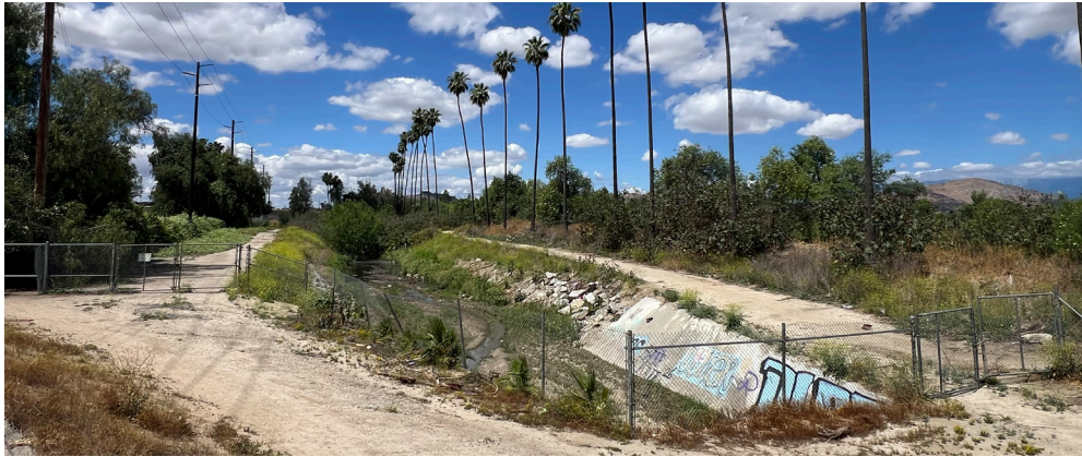
2. Drainage channel along north edge near entrance.
