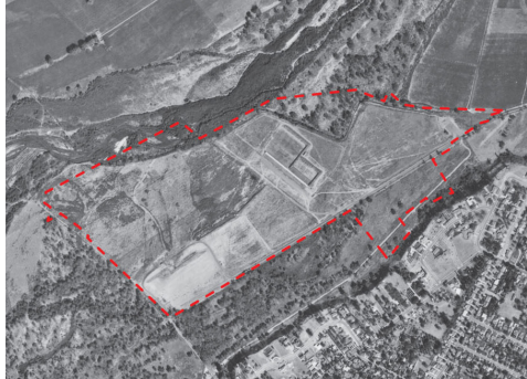
1959: trench and fill operations buried waste up to 15 feet below grade. The Santa Ana River has been diverted and no longer crosses the west side of the site.
