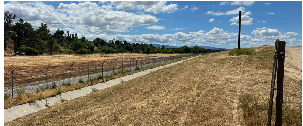
4. Swale, fence and bike path along S edge of mound.
