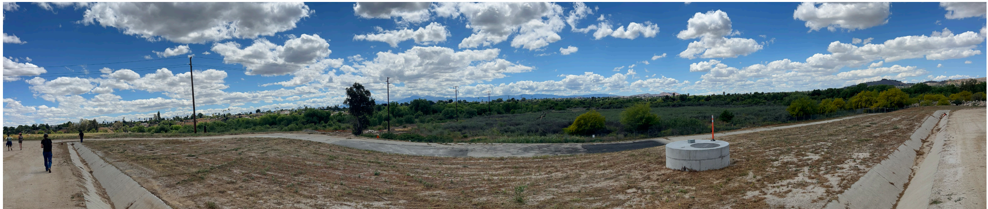
3. Service road ramp, manhole and river valley view from west edge of mound.
