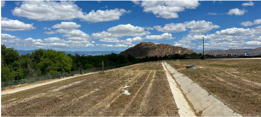
1. Drainage swale and methane cap at top of northern slope.
