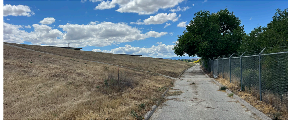
4. Service road along north edge looking west.
