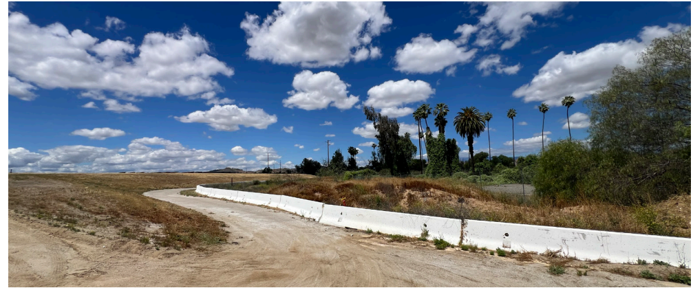
4. Service road along north edge near entrance.
