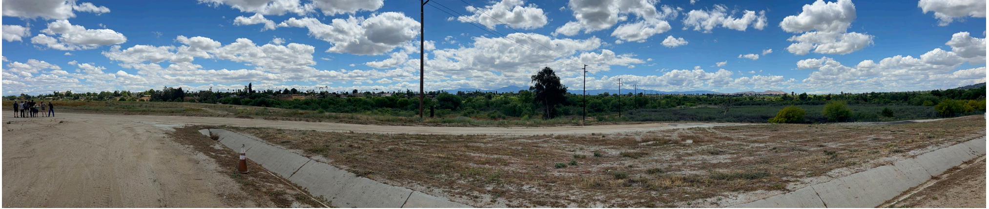
2. Drainage channel along west edge above service road ramp.
