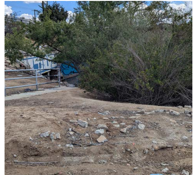
5. Culvert and concrete walkway with metal railing and debris pile
