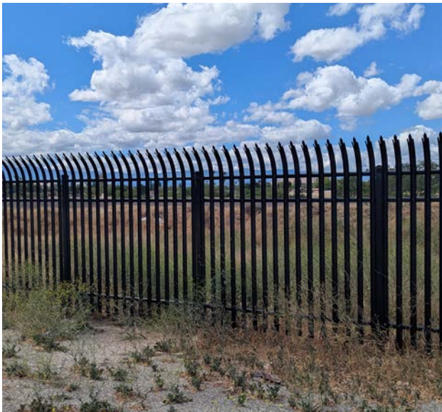
4. Fence barrier, looking west
