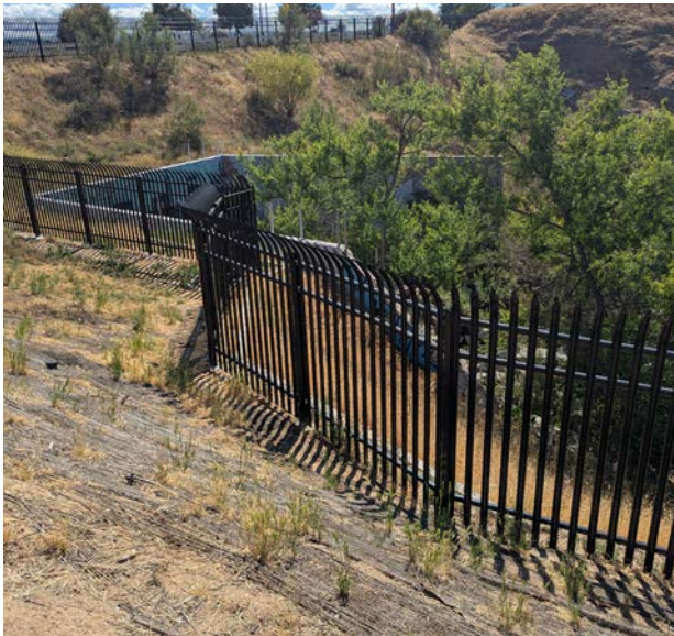
4. View from car wash down into creek and culvert
