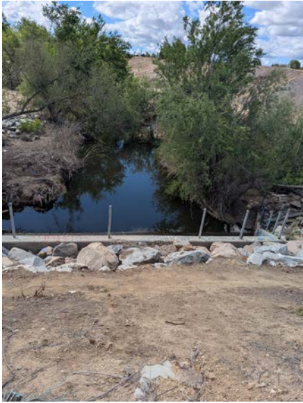
1. A large culvert with debris in the background
