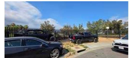
Storm Drain right near edge
