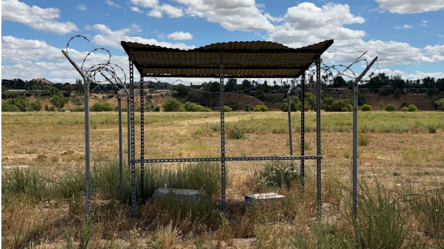
Brutal shade structure
