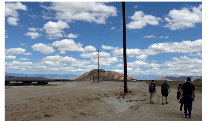
Above ground electrical poles
