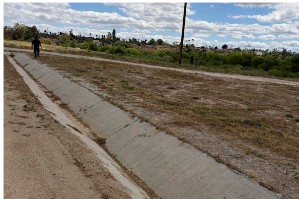
Culvert to divert water
