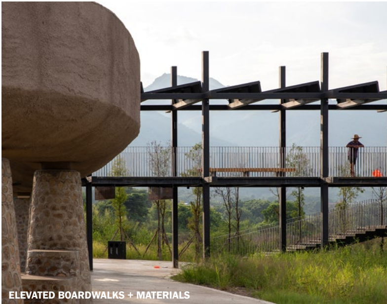
ELEVATED BOARDWALKS + MATERIALS
