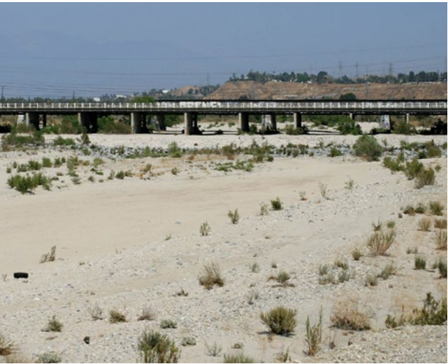
View upstream from the site, a typical sandy, dry, alluvial wash with alluvial scrub plants. Mission Bridge stands in the background, providing access between Riverside and Jurupa.
