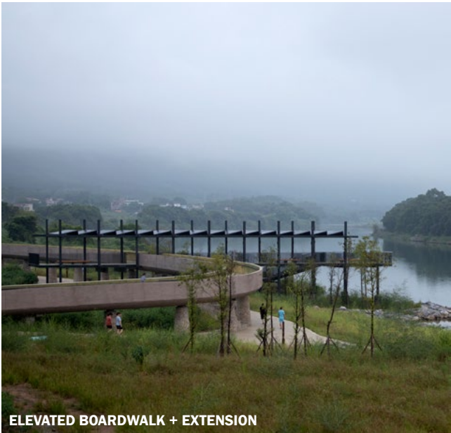
ELEVATED BOARDWALK + EXTENSION
