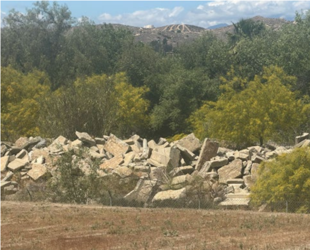
Rock levee as seen from top of Solar Farm vantage point, protecting landfill integrity from flood damage.
