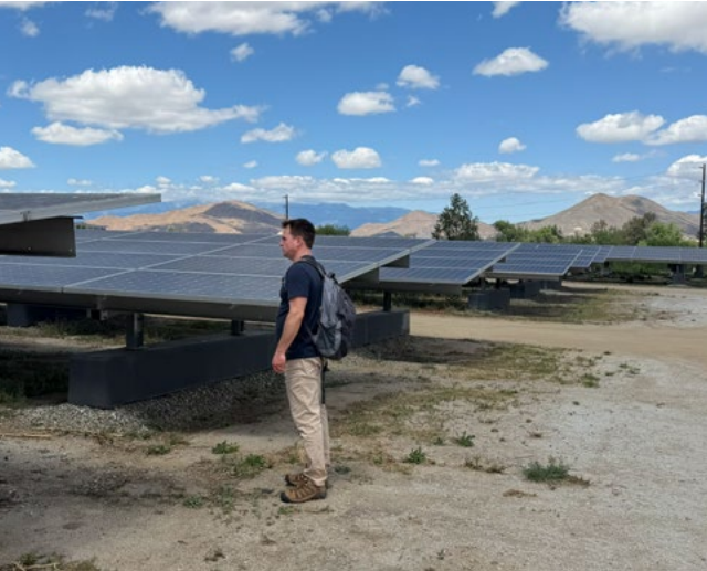
Close up of solar panel farm on top of landfill. Jurupa Hills in the Background, and San Gabriel Mountains in the distance.
