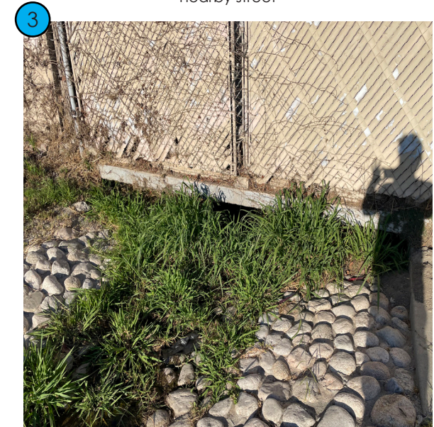
End of concrete and cobble swale. Water leads to next street and eventually to drainage
