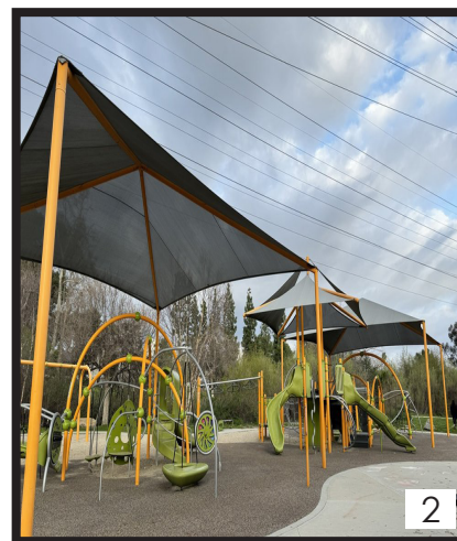
Shade Structures over Playground
