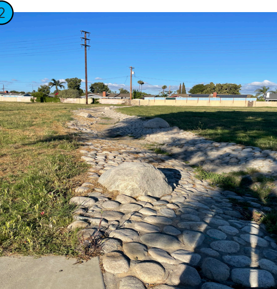
Concrete and cobble swale with some large boulders going through turf field
