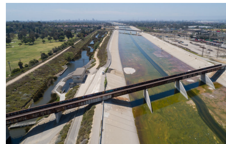
Dominguez Gap Wetland Pump Station 14
