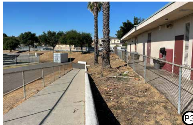
2nd-6th grade back side classrooms near path to recess area
