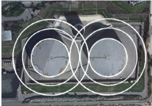
The pair of 220-foot diameter fuel tanks pre-demolition.
