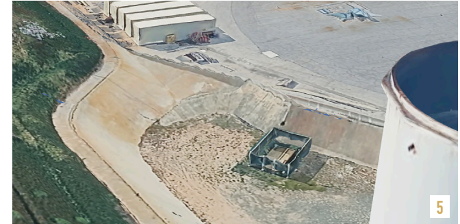
(5) Potential amphitheater site with fuel tank backdrop.
