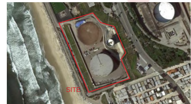
Tanks in process of demolition, 2011. North tank removed, south tank still standing. (Image: https://earth.google.com/ )
