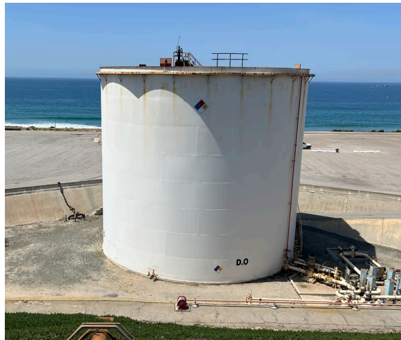
Tank current condition.
