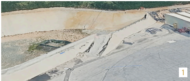
(1) Steep concrete banks in fair condition for roller sports.
