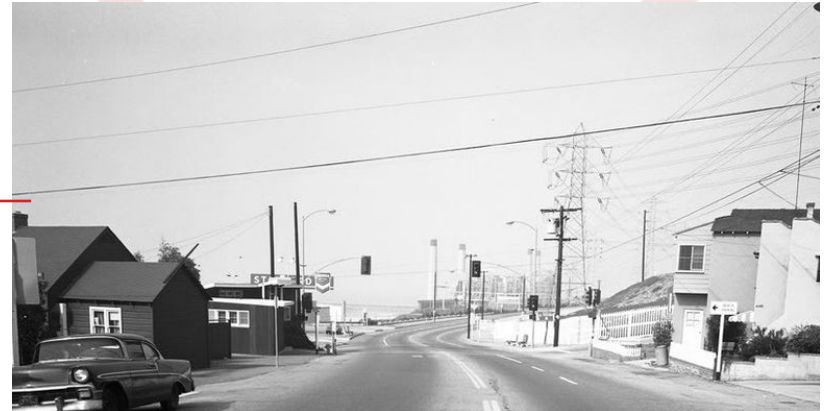
1950s view from Vista del Mar Blvd. looking north towards the El Segundo Power Plant and Chevron gas station adjacent to the site (Photo: www.osoport.com )
