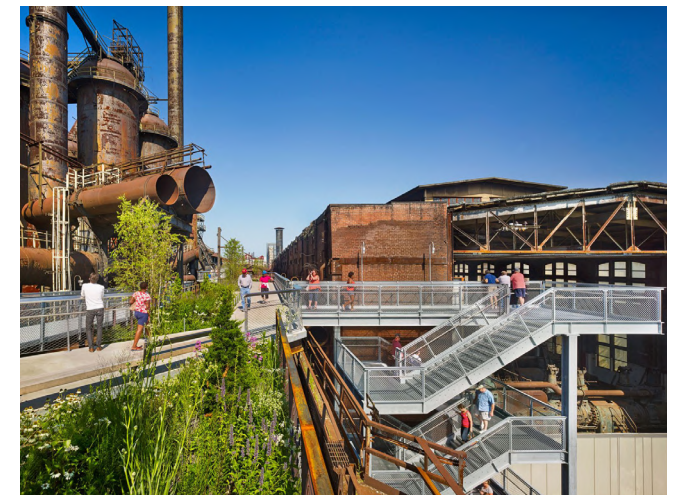
Hoover-Mason Trestle, former Bethlehem Steel Plant, PA (Photo: https://www.wrtedesign.com/projects/hoover-mason-trestle )
