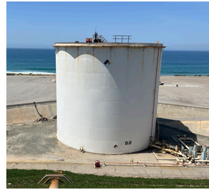
Tank current condition.
