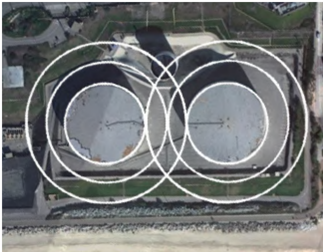
The pair of 220-foot diameter fuel tanks pre-demolition.
