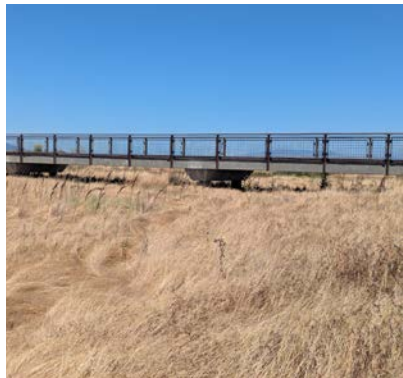
Bridge over future creek
