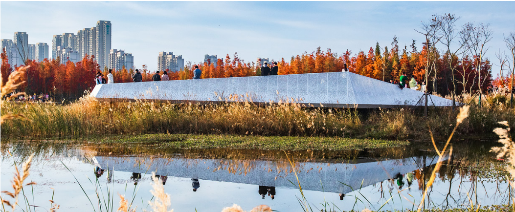
Bridges and platforms for birding - Kongjian Yu, Turenscape
