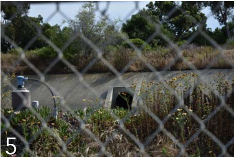
SeaWorld Stormwater Detention Basin
