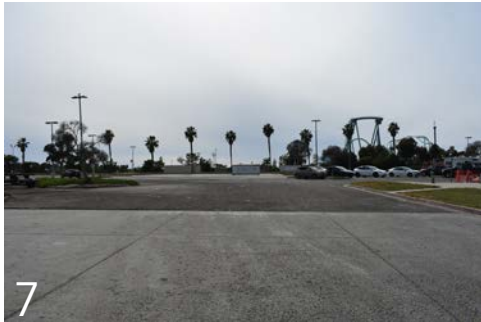
South Shore Park Parking Lot
