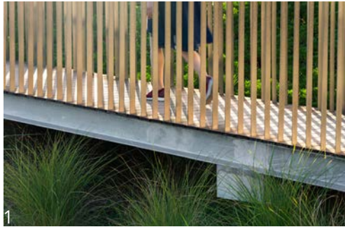
1 Wood & Metal Boardwalk
