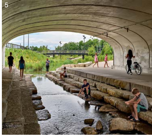
Creek Daylighting & Access
