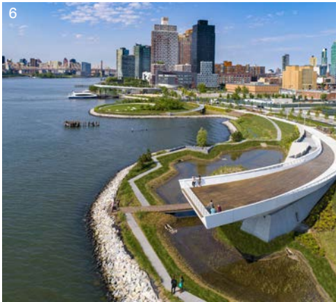
Constructed Wetland & Overlook
