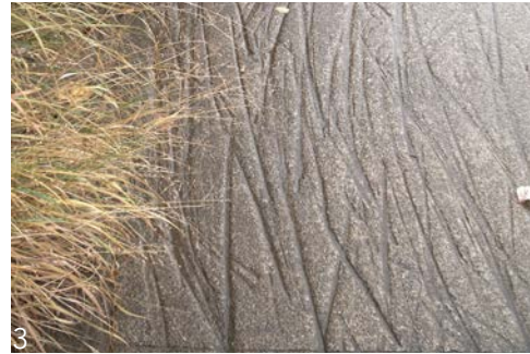
3 Etched Concrete Paving
