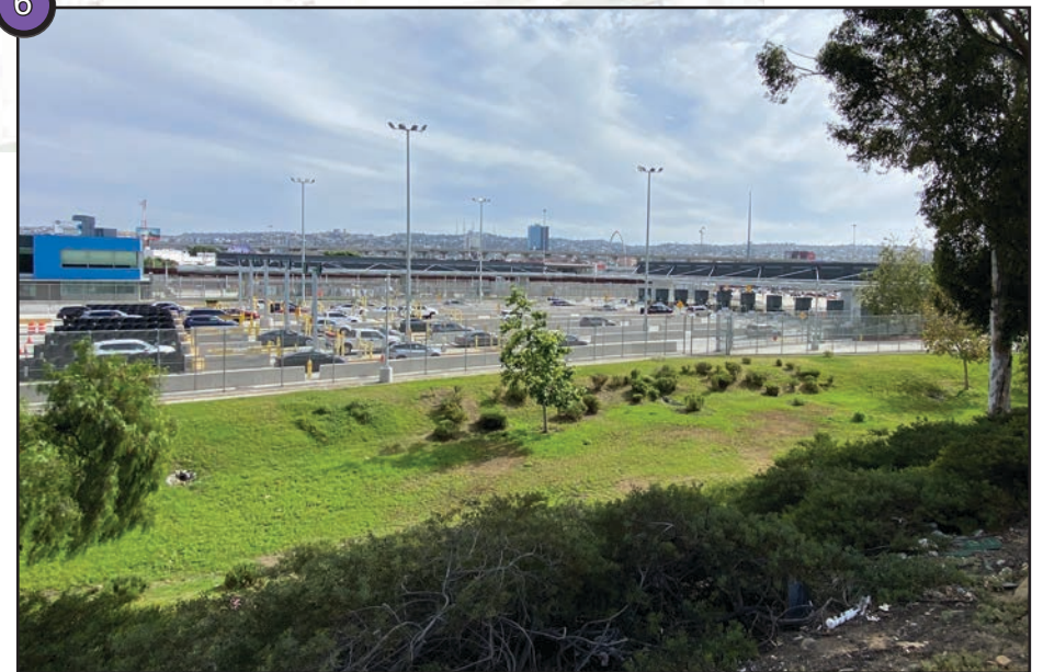
View of vehicular border crossing lanes over irrigated swale
