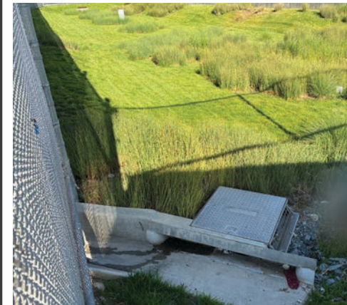
This drain on SW part of site leads to a bioretention basin
