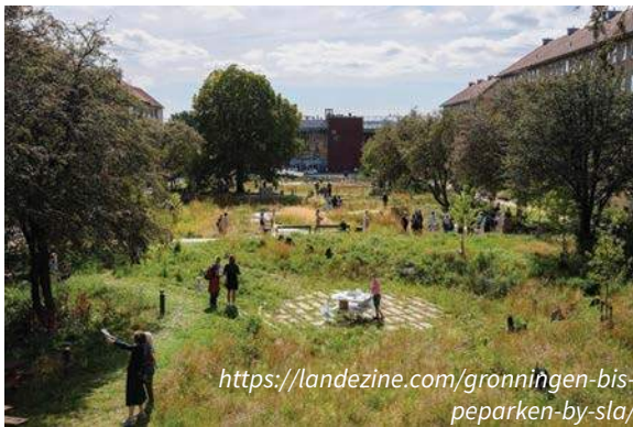
Example: Multi-use infiltration basin-dry weather
