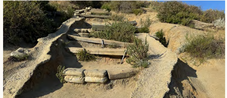
1. Erosion cuts around steps along the existing trail.
