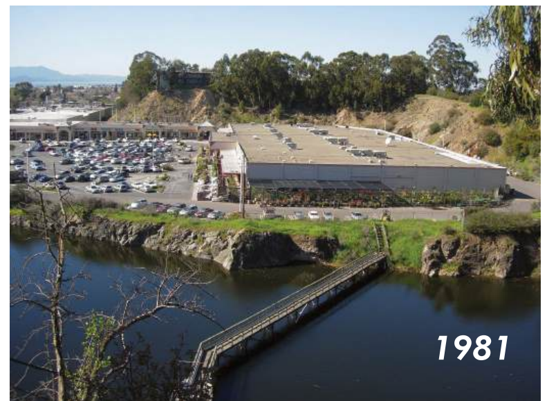
Prior to recent redevelopment of the site, the quarry reservoir remained unfenced
