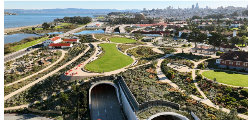
Park built over 7-lane highway
