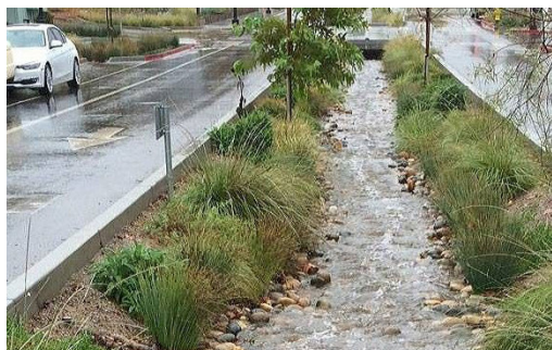
Rain Garden along street to filter stormwater
