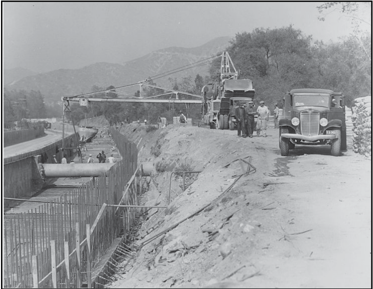
VERDUGO WASH AT GLENOAKES WPA Era Channelization 1936
