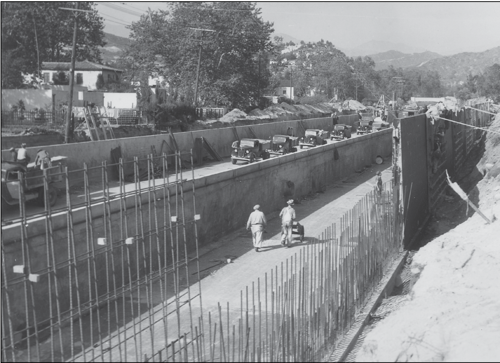
VERDUGO WASH AT GLENOAKES WPA Era Channelization 1936
