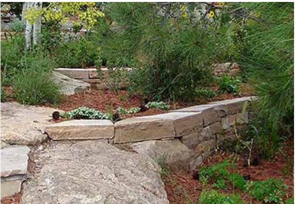
Stack Stone Terrace Wall
